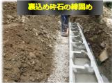
裏込め砕石の締め
