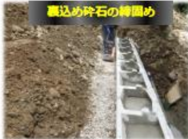
裏込め砕石の締め
