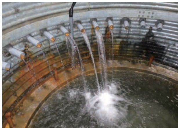
(集水井工坑内集水状況)
